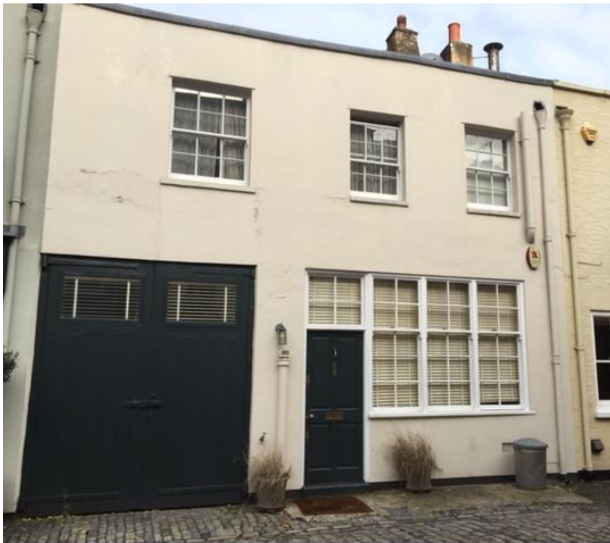
Front Elevation of Application Site
