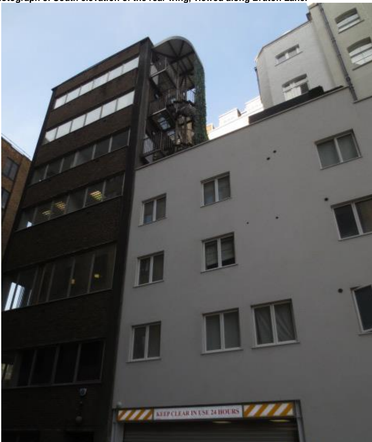
Photograph 3: South elevation of the rear wing, viewed along Bruton Lane.
